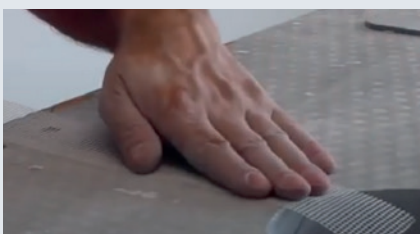
1 Placer SkamoEnclosure Joint Tape.
